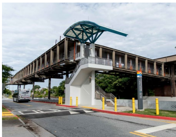
Reynoldstown Bridge: Before and After
